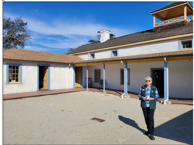
West courtyard of the Casa de Dana
