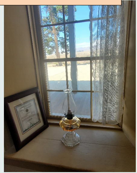
Window showing thickness of adobe
